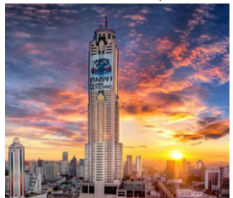
Baiyoke Tower II
